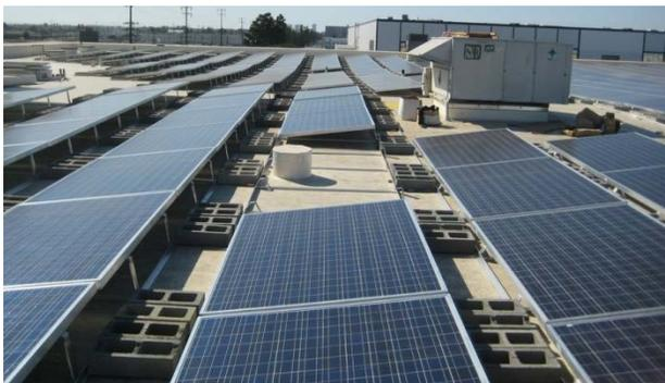
**THIS IS AN EXAMPLE OF A BALLASTED SOLAR ARRAY ON A LARGE FLAT ROOF. CONCRETE BLOCKS PRESS THE METAL RACKING TRAYS DIRECTLY AGAINST THE ROOF MEMBRANE. NOT ONLY IS THIS A BAD IDEA FOR THE ROOFING SYSTEM, THE BIG RED FLAG HERE IS WEIGHT. IN A HEAVY RAIN THE WATER CANNOT FLOW TO THE DRAINS AS DESIGNED, PUTTING THIS ROOF IN SERIOUS RISK OF COLLAPSE.**
