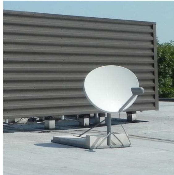
**A SATELLITE DISH IS MOUNTED USING CONCRETE BLOCKS AS BALLAST. THE BLOCKS ARE RETAINED BY A METAL TRAY WHICH SITS DIRECTLY ON THE ROOF MEMBRANE, LEADING TO PREMATURE FAILURE. IRONICALLY, IN THE BACKGROUND IS A BEAUTIFUL ROOFSCREEN WITH PROPERLY INSTALLED AND ROOFED ATTACHMENTS.**
