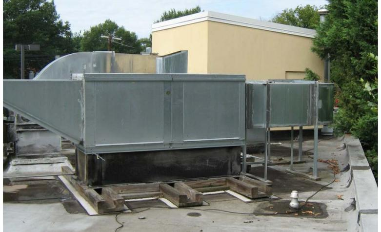
**THIS HVAC EQUIPMENT, INCLUDING SOME LARGE ELEVATED DUCTWORK SITS UNDER ITS OWN WEIGHT ON REDWOOD SLEEPERS. WATER IS RESTRICTED FROM FLOWING TO THE DRAINS WHICH CAUSES PONDING AND A BUILDUP OF MUD AND DEBRIS.**
